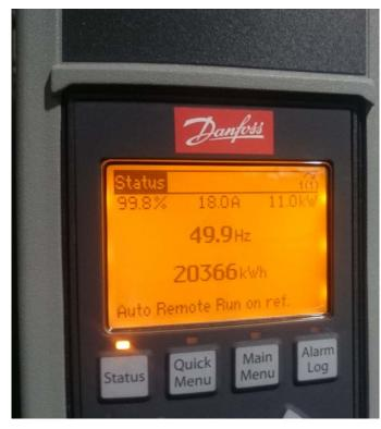
Pump Speed and Consumption before VSD Installation
