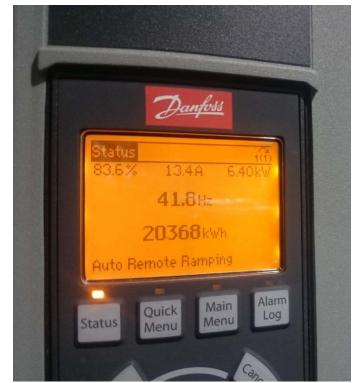
Pump Speed and Consumption after VSD Installation
